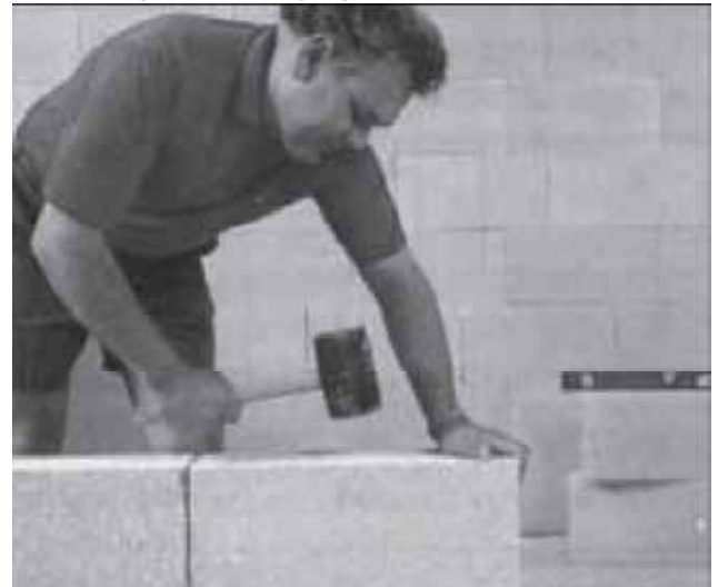
Figure 6.4 – Laying Blocks
