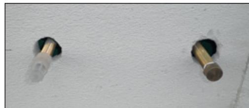
Figure 3.3.2 Neat finishes of installed services
