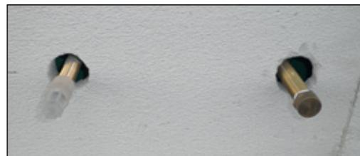
Figure 3.3.2 Neat finishes of installed services
