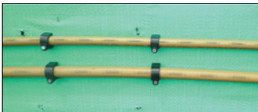
Figure 3.3.1 Installed piping services prior to the installation of Hebel PowerPanelXL
