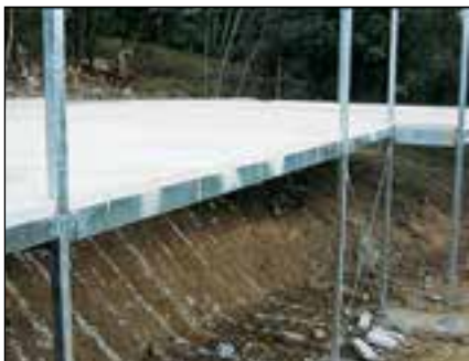
Fig 1.1 Residential Suspended Ground Floors
