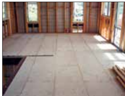
Fig 1.2 Residential Suspended First Floors
