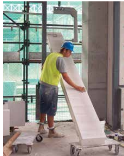
Fig. 5.3 Vertical panel lift attachment.
