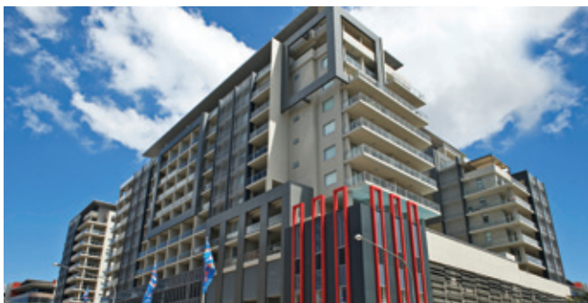
PowerPanel – Builder/ Developer: Casumo Constructions; Architect: BD Architecture
