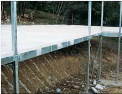
Fig 1.1 Residential Suspended Ground Floors
