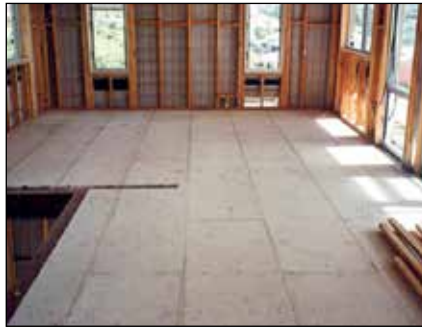
Fig 1.2 Residential Suspended First Floors
