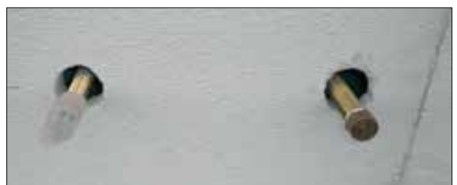
Fig. 3.3 – Neat finishes of installed services
